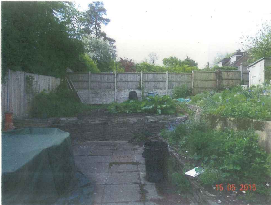
Scale: Veg plot wall 4' 6" high Retaining boundary wall 3' high Fence panel 4' high x 6' long
